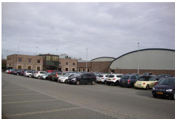
Bebouwing health center 'Pellikaan'
